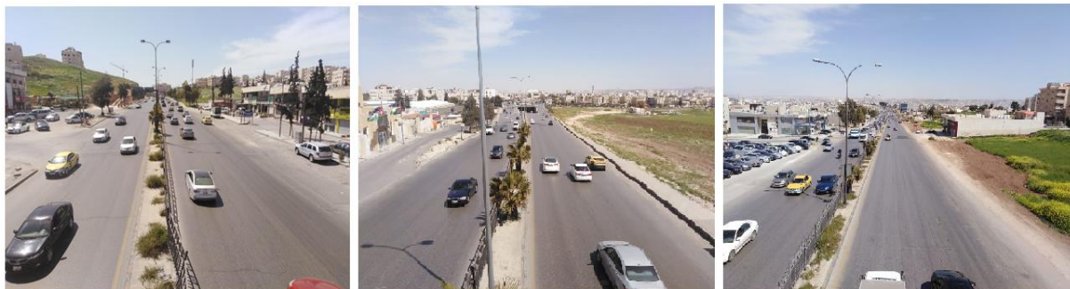
Figure 2 Lanes of Alhizam Highway (Panoramic view)
