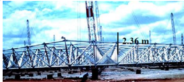
Figure 2 Trusses bolted on the ground [3]
