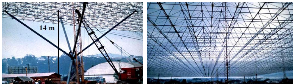
Figure 3 Structure lifted at the final level [3]
