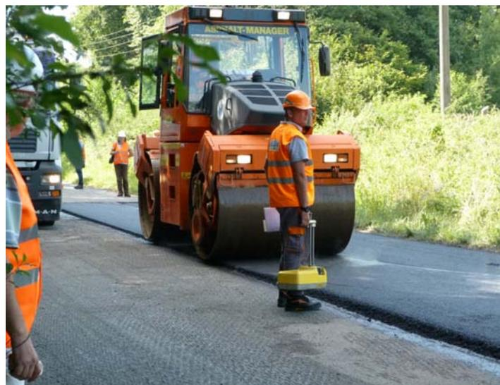
**Figure 3. Compacting the layer and density control**
