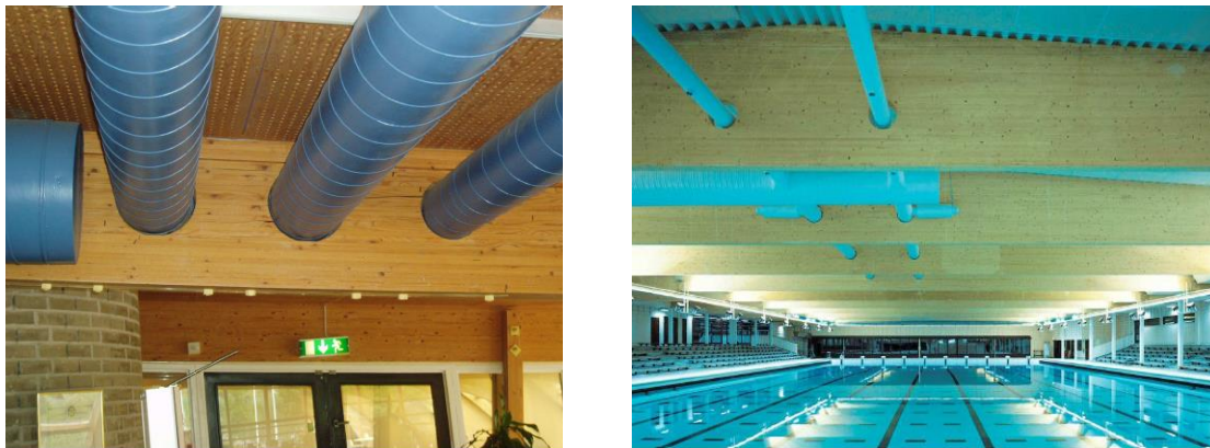
Figure 1 Glulam beams with openings [1]
