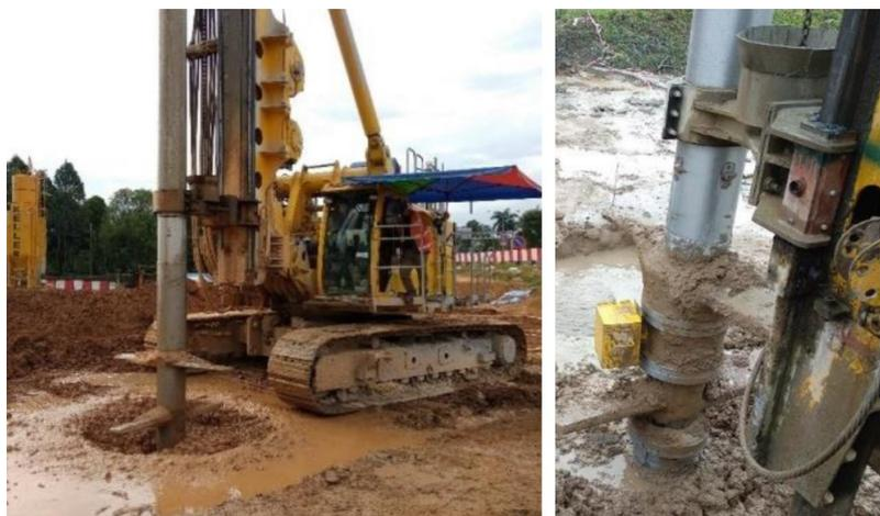
Figure 2 Application of wet DSM [40]
